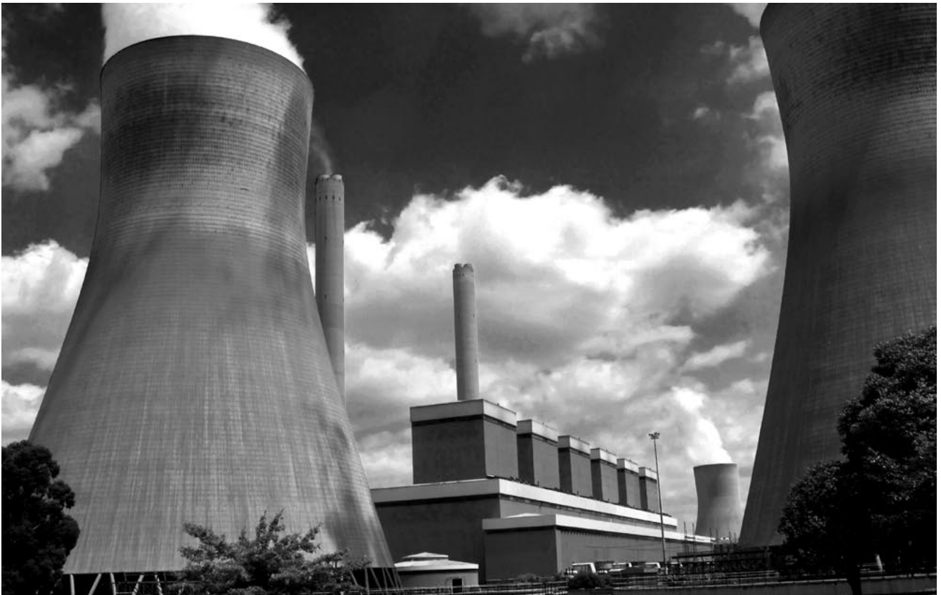
Eskom's Duvha power station, east of Witbank, Mpumalanga
